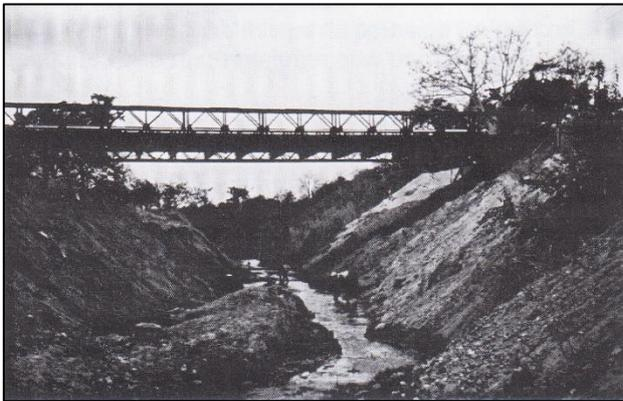
All was not over, but things moved fairly smoothly as the end dams were cast, a culvert was put in the approach road, the road was brought up to level, the wearing surface was laid and the banks were landscaped and compacted by local labour, leaving the bridge ready and the project finished in good time for the official opening on 31st March.
